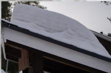
Remove snow accumulations from the roof before the snow reaches 50% of the "safe" maximum depth. Do not send employees onto the roof once the snow load approaches the live load capacity. Remove snow during a storm only if the forecast indicates that the total snowfall will result in dangerous accumulations.
